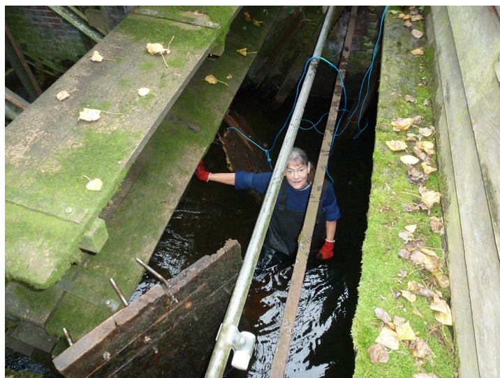
Claire can be seen here clearing the broken wood of the sluice gate from the waterwheel.
